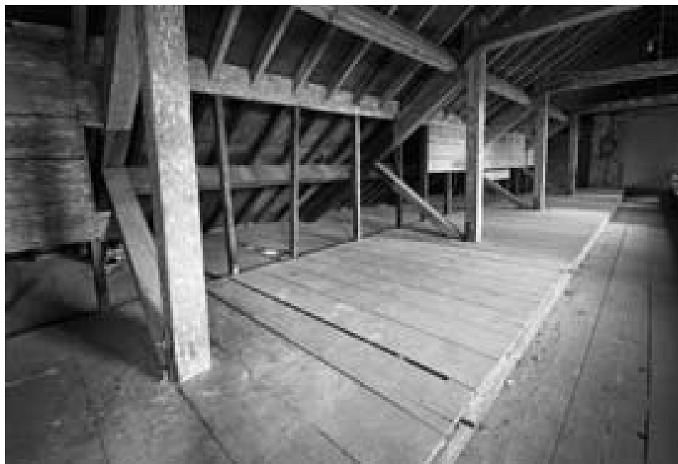
Armagh Workhouse, The sleeping platforms under the slates on the third floor.
