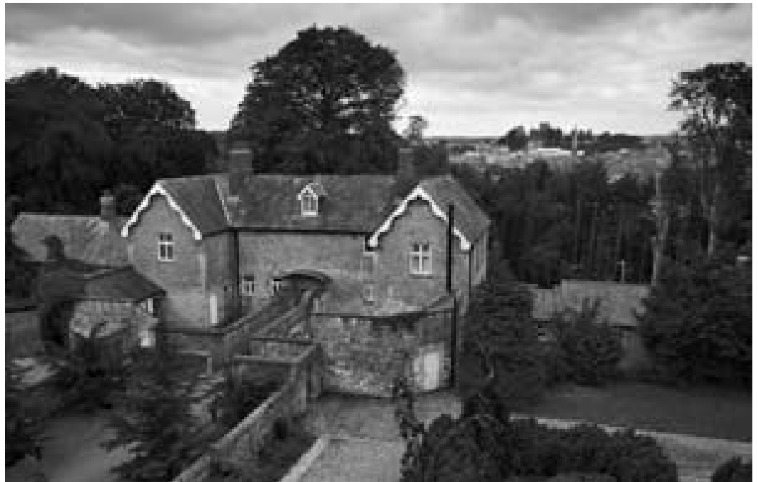
Armagh Workhouse, The front building seen from the third floor dormer window of the main building.
