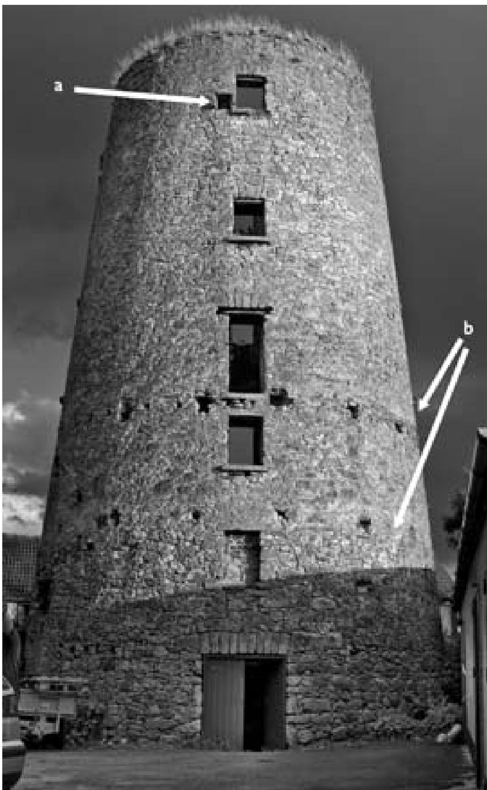
fig 6. The north face of the windmill showing A: opening for fan and B joist holes for Reefing Stage level and supports.
